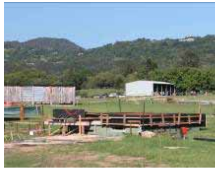
Lot 105 featuring inground water tanks
